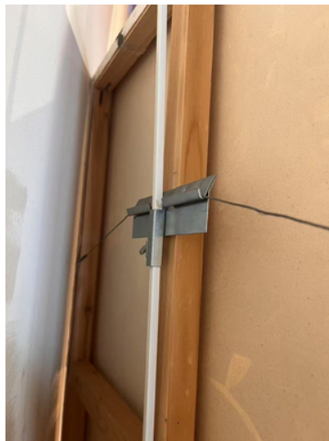
Hi-Holder + V/D/Eye hook + Hanging Wire
